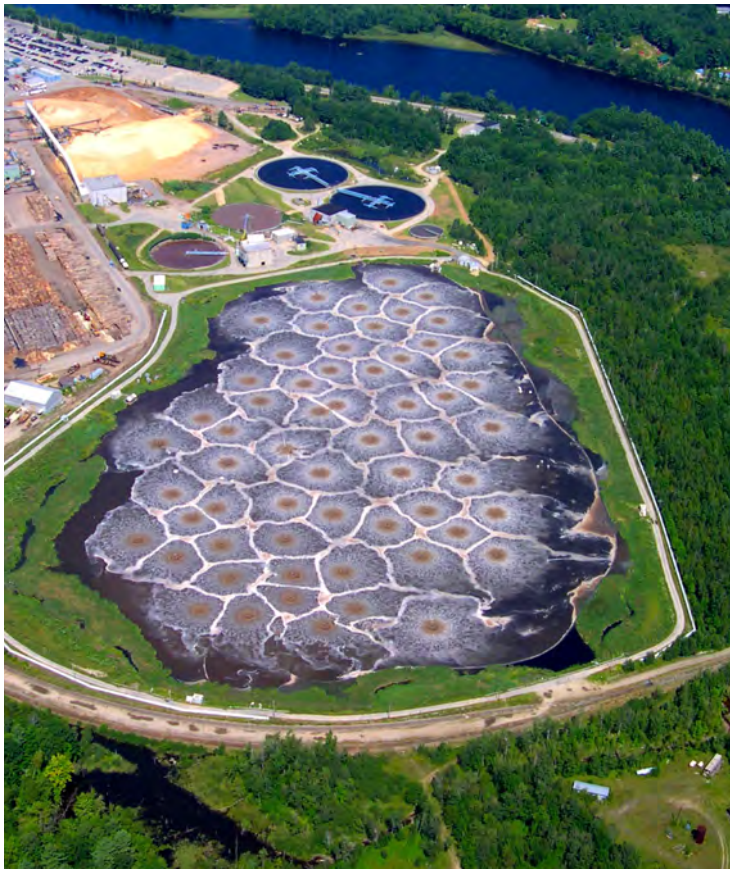
Pulp mill lagoon wastewater headed to the Androscoggin- Photo: Point of View Helicopter Services
