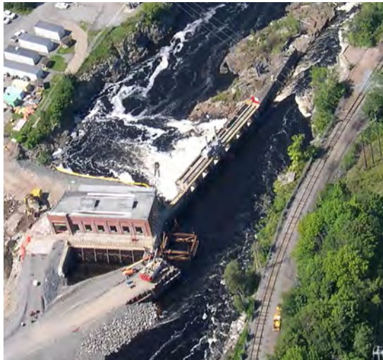
Beginning of Milltown dam removal, USA on right, 2023
