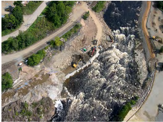
Dam removed, USA on left, 2024
