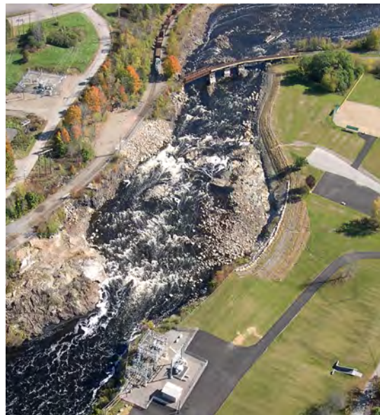
Site restoration underway, Canadian side seeded and ball fields, 2025
